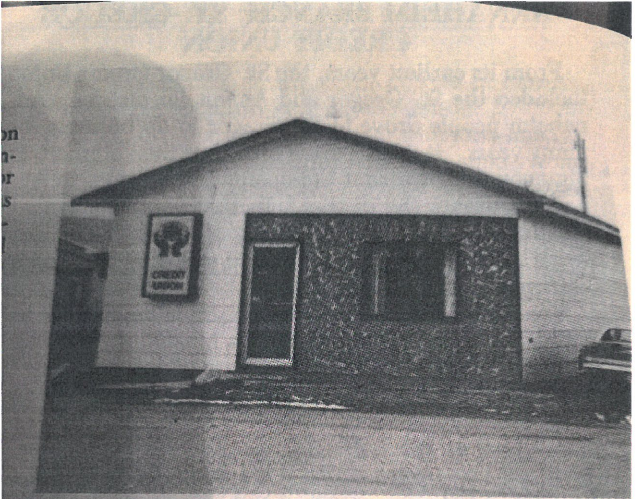
Anaheim Credit Union Office.
